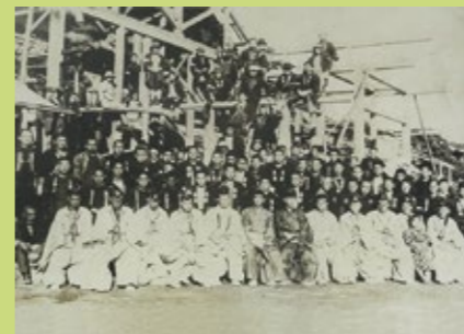
In December 1935, laying the roof festival of Togoku Keishin Dojo was held. (Shinto priest and the leaders of craftsmen line up in the front row. There are about 80 craftsmen in the back.)
